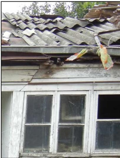
***Broken and leaking asbestos roofs:*** Because of heavy rains and lack of maintenance, the roofs of many Armenian houses are severely deteriorated - slates are often broken, and rainwater leaks in. Besides, most roofs are made of asbestos, which is a hazard for the health of the residents. Fuller Center replaces broken asbestos roofs with corrugated tin roofs on timber frameworks.
